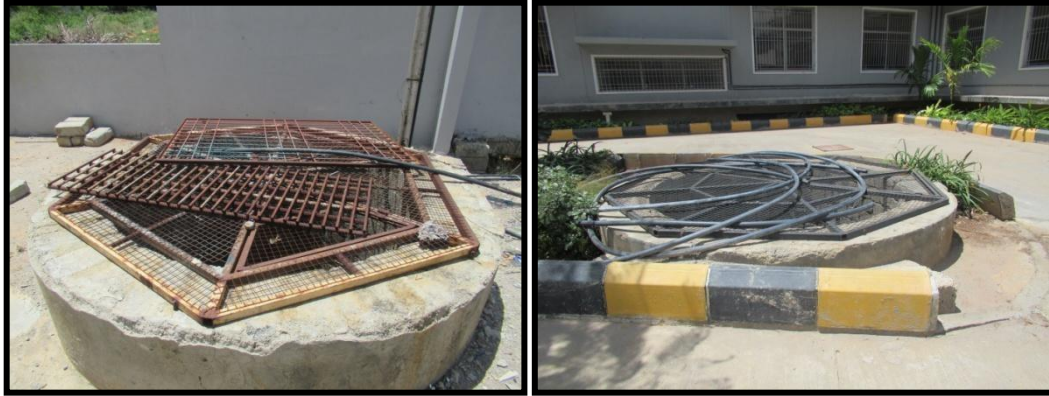
Fig: Rain Water Harvesting Pits
