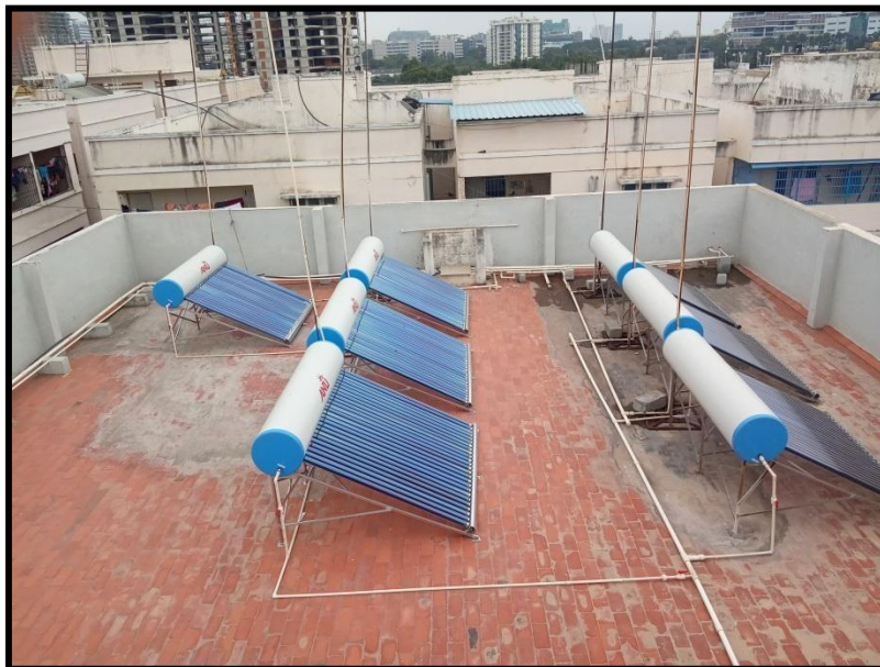
Fig: Evacuated Tube Collector (ETC) Stainless Steel 250 LPD
